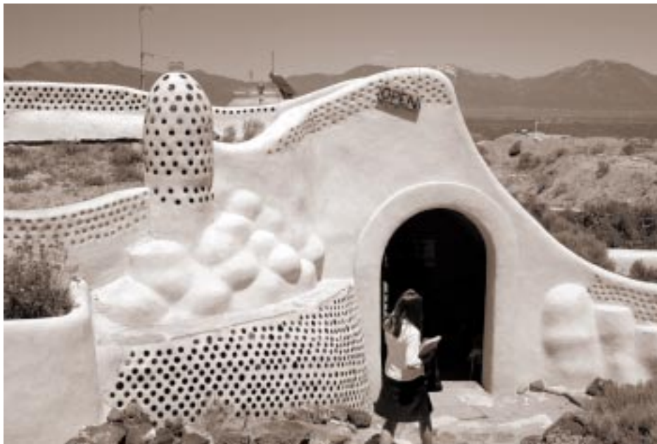
A visitor enters the west side of a model Earthship open to the public (above) near Taos, NM. Recycled bottles are embedded in the adobe wall, which is built with used tires. The south wall (top) provides solar electricity, light and winter heat. More conventional styles are possible.
